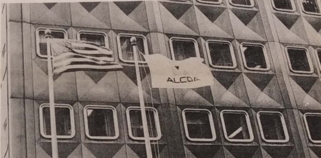
Alcoa Corporation Headquarters in Pittsburgh another multi national corporation that exploits the people.
